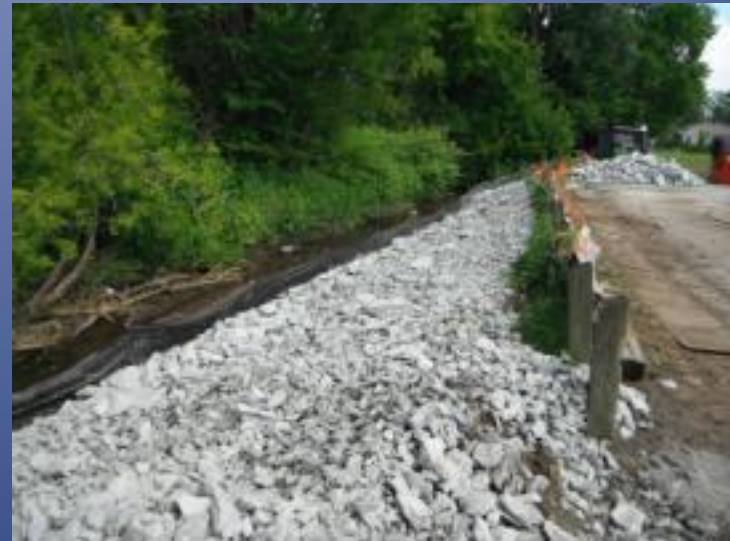
Stevens Brook- runoff and soil retention measures, rip rap, & geo-fabric
