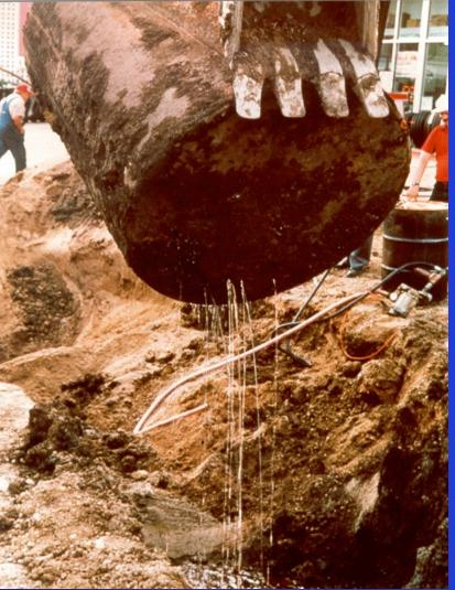
A leak from an underground gasoline storage tank releases a single product which first saturates the adjacent soils and then migrates into groundwater. Following the groundwater gradient . . .
